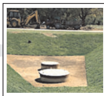
Creating a sunken area around the Porous Composite Concrete recharge system.
